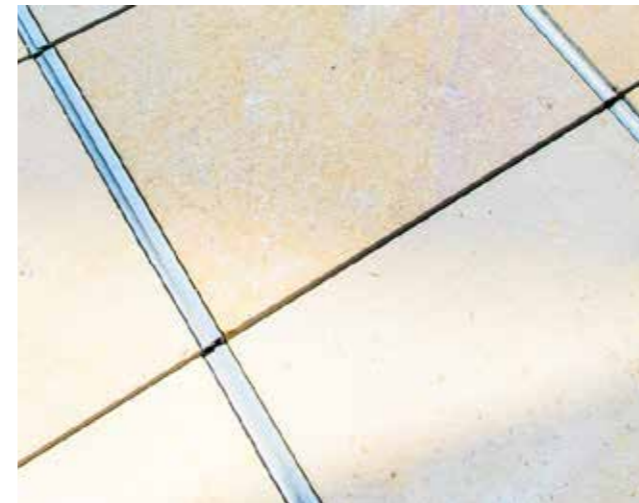
Joint de dilatation
